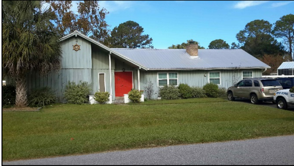
Drainage ditch visible in yard
