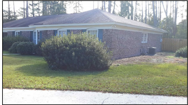
HVAC at grade
