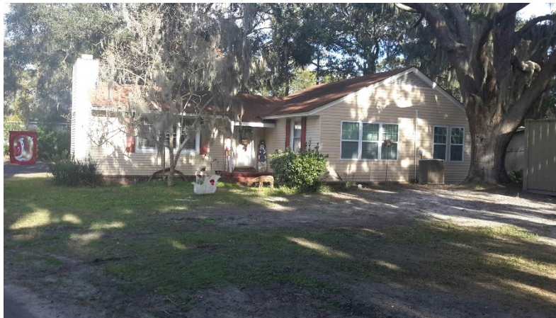
HVAC unit not elevated
