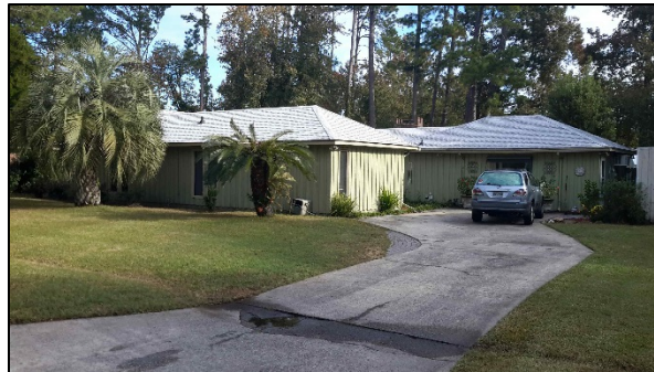
Drainage ditch visible in yard
