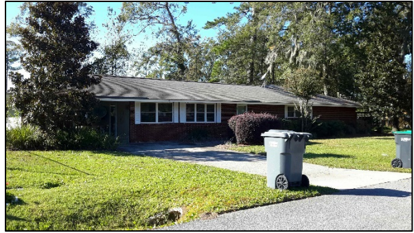
Drainage feature in yard
