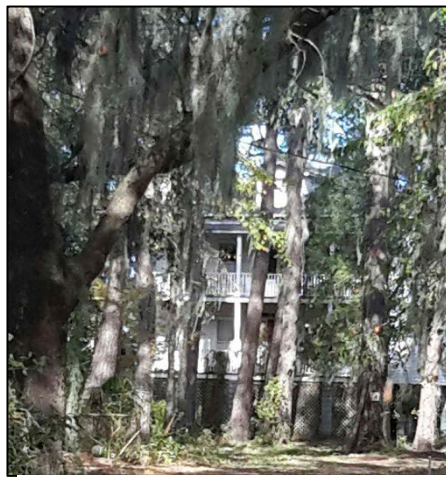
Home elevated on piers
