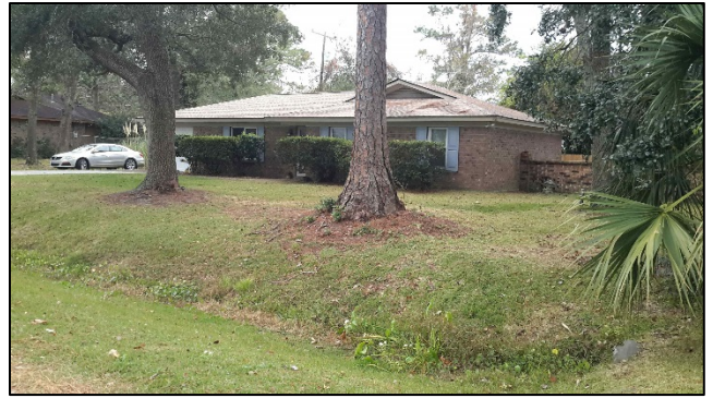
Drainage feature in yard
