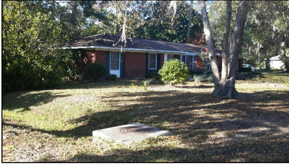
Drainage ditch adjacent to home
