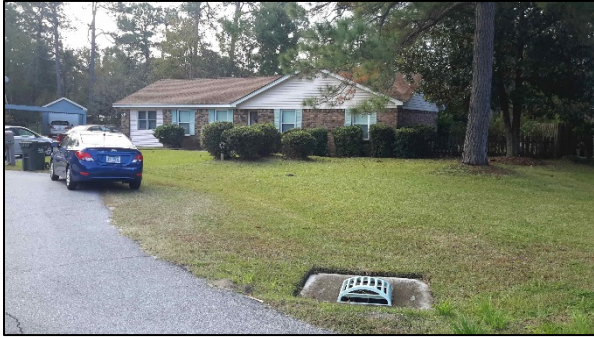
Stormwater inlet visible in yard
