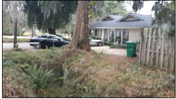
Drainage feature in yard
