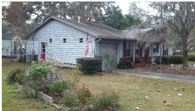
HVAC at grade
