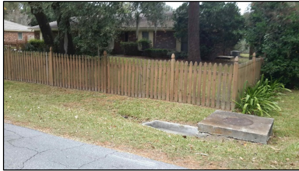
Drainage feature in yard
