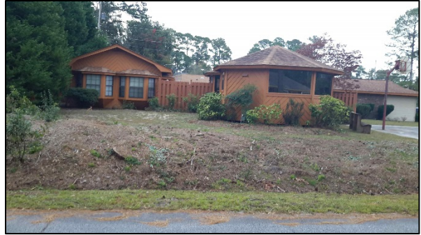
Drainage feature in yard
