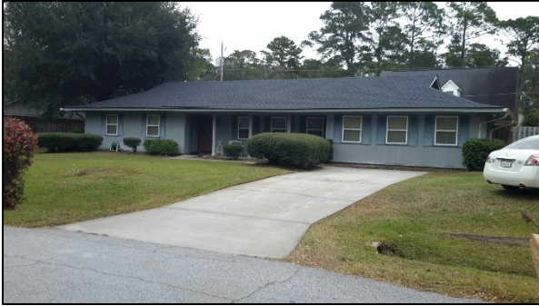
Drainage feature in yard
