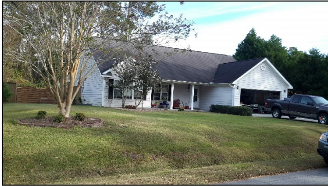
Drainage feature in yard
