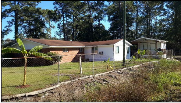
Elevated secondary structure
